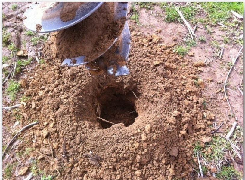
Figure 4. Our rough hole made by a modified auger.
